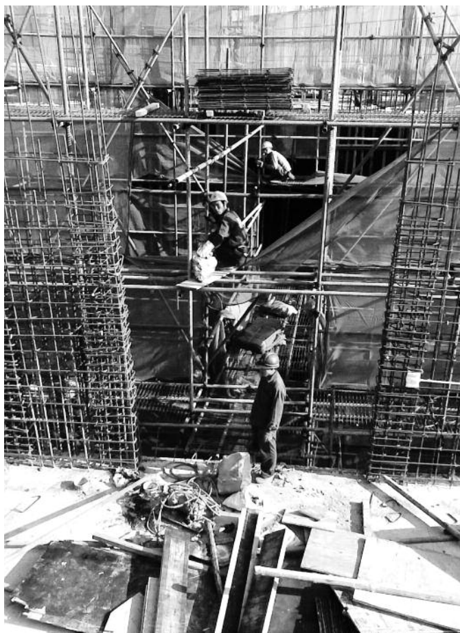
Workers on a construction site
