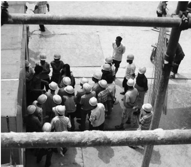
Workers on struggle at construction site
