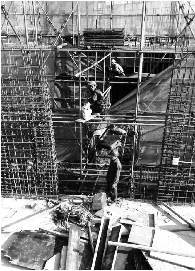
Workers on a construction site
