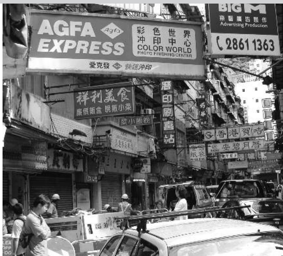
Wedding Card Street before demolition
