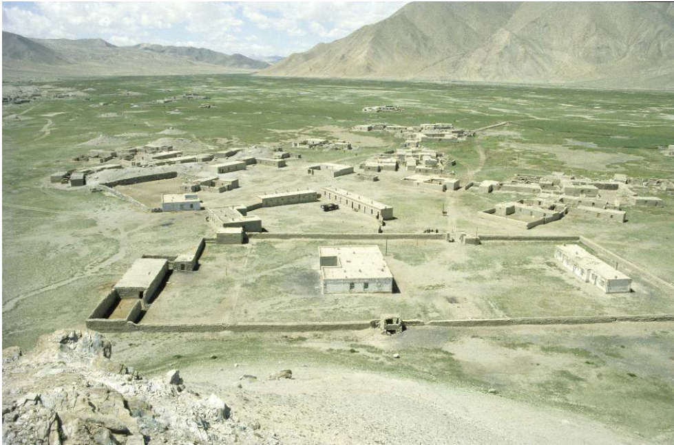
Photo 3. The settlement of Subashi as the production brigade's centre for infrastructural assets
