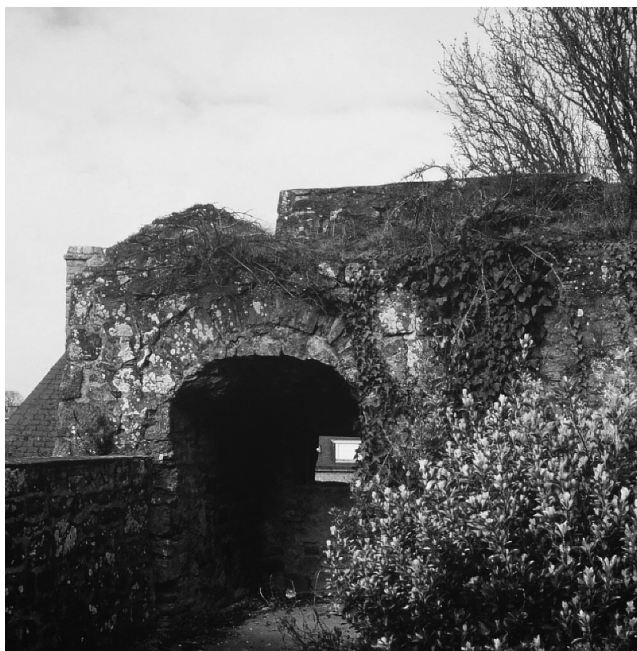
Figure 2: Actual remains of Avranches' keep. Figure 2: Vestiges conservés du donjon d'Avranches.
