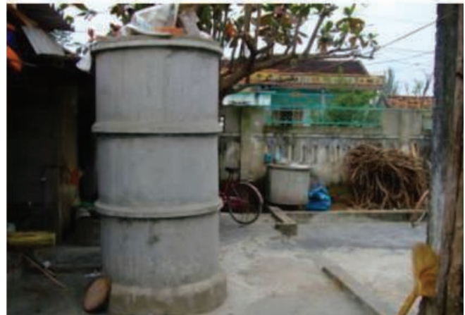
Figure 4. Typical box tank from Nam Dinh Province (top) and typical cylindrical tank from Nghe An Province
