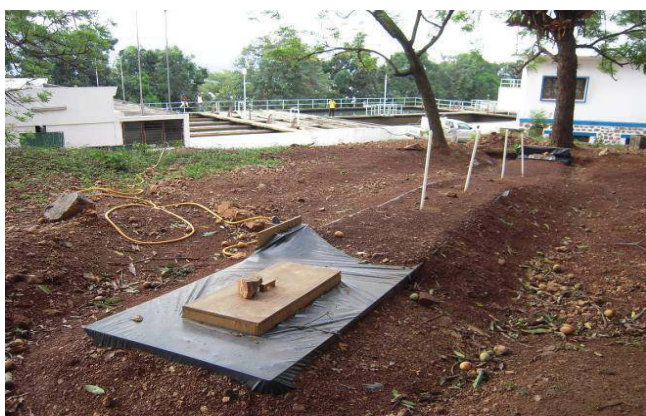
Figure 1c. View of the completed pilot (supply hatch, the 4 piezometers, and the receiver)
