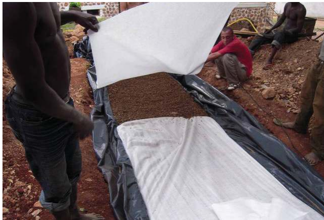
Figure 1a. The trench in which the pilot was built
