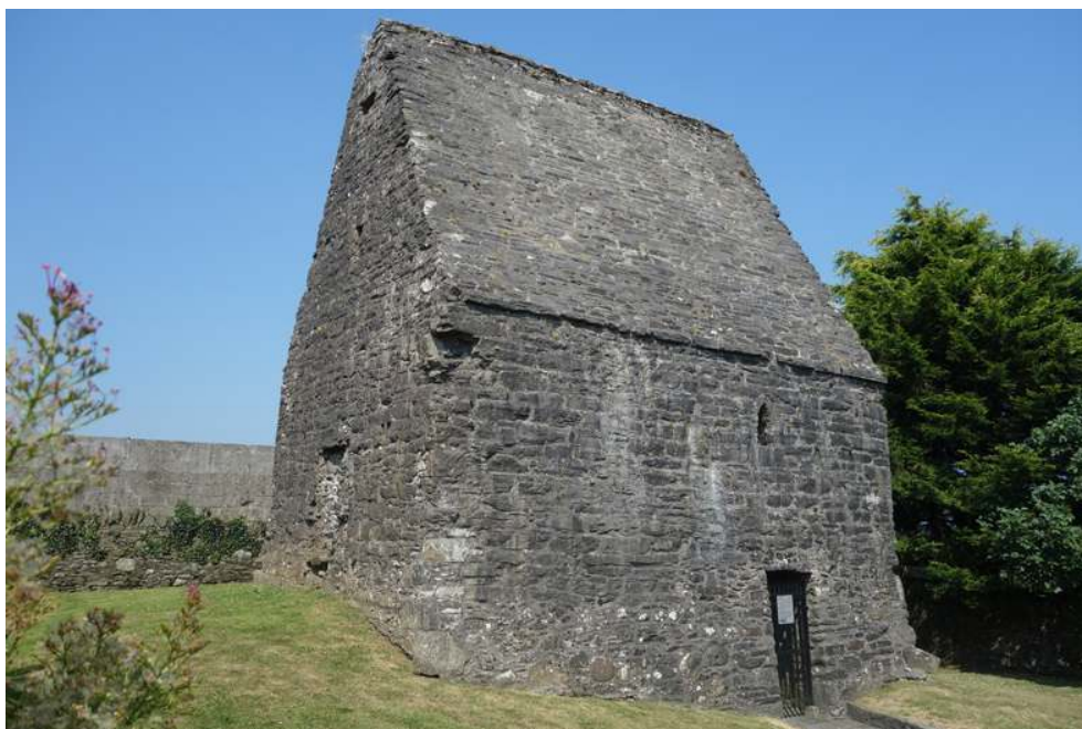
Fig. 3 – St Columba's House, Kells. This late eleventh century church appears to have been part of a complex, within the monastery of Kells, associated with care of the sick (Photo T. Ó Carragáin).
