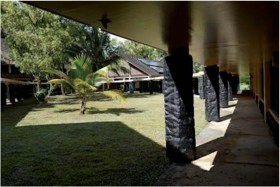
PHOTO 1. – The FSM national capital complex in Palikir, Pohnpei, constructed in the 1980s, incorporates materials replicating the natural basalt columns used in the structures of Nan Madol, an ancient political center on Pohnpei, thus visually integrating traditional Micronesian forms with those of constitutional government (picture by the author)
