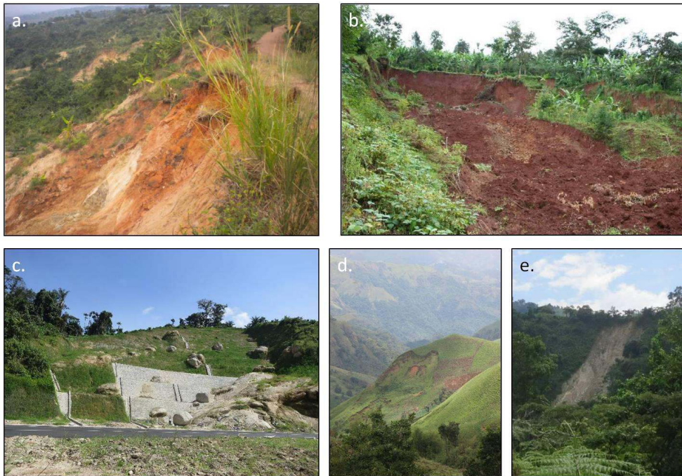
A) DEEP LANDSLIDE SCARP (AND SEVERAL IN THE BACKGROUND) IN THE LOWLANDS OF KATUMBA PARISH, BUNDIBUGYO DISTRICT, RWENZORI MOUNTAINS (UGANDA); B) 8M DEEP TRANSLATIONAL LANDSLIDE REACTIVATED IN SEPTEMBER 2014; BUSHYI SUB-COUNTY, BUDUDA DISTRICT, MT ELGON (UGANDA); C) LANDSLIDE OF MARCH 2014 STABILIZED WITH TERRACES AND RETAINING WALLS ALONG THE BAMENDA – MAMFE ROAD, CAMEROON; D) SMALL SHALLOW LANDSLIDES WITHIN A LARGER LANDSLIDE, MAGHA, BAMBOUTOS CALDERA, WEST REGION, CAMEROON; E) DEBRIS SLIDE INTO NYAMWAMBA RIVER, KILEMBE SUB-COUNTY, KASESE DISTRICT, RWENZORI MOUNTAINS (UGANDA).
