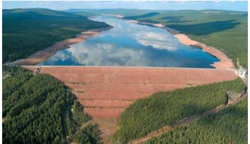
The Trångslet Dam in Sweden (photo: ICOLD)
