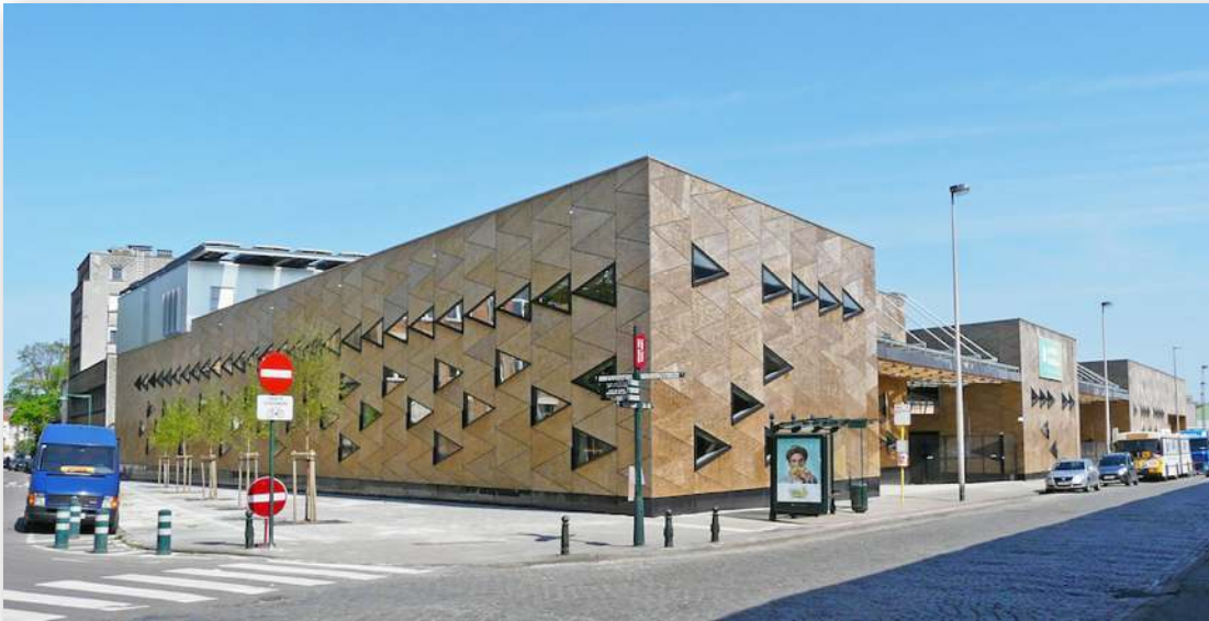
Figure 7. “Economic expansion” part of the Tivoli sustainable neighbourhood. Greenbizz building composed of a green business incubator, offices and production workshops. Elaborated by the firms Architectes Associés, Setesco (stability), Istema - FTI – Cenergie (special techniques), Daidalos Peutz (acoustics). Source: Architectes Associés
