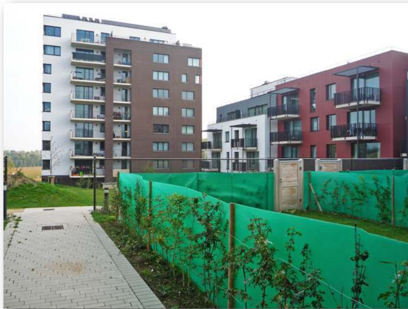
Figure 8. Rue Bruyn project – Bruyn North site: screens placed along private gardens. Source: photo by A.-L. Wibrin
