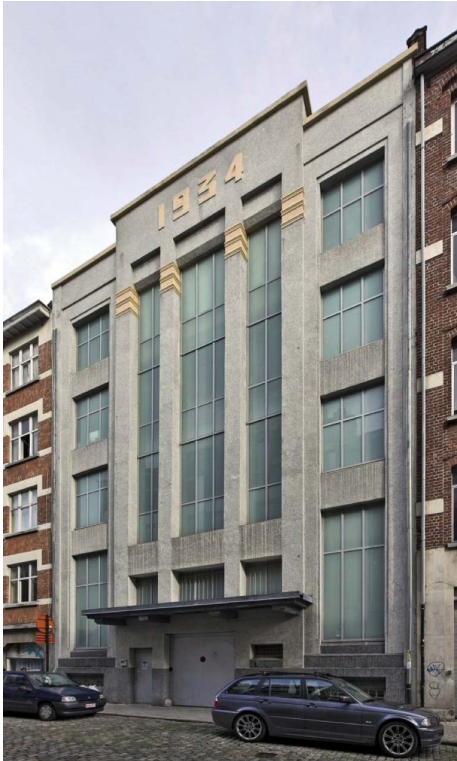
Figure 9. The façade of the textile warehouse Etablissements I. & M. Blum (1934) makes use of cimorné 14 interwar decorative cement render
