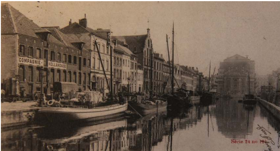
Figure 2. Nineteenth century view of the Brussels docks. On the left, the hay warehouse (1841) of the Ancienne Compagnie Hollandaise with two pulleys with protective hood, and tiers of doors to lift the hay inside the building. Quai au Foin 59-60
