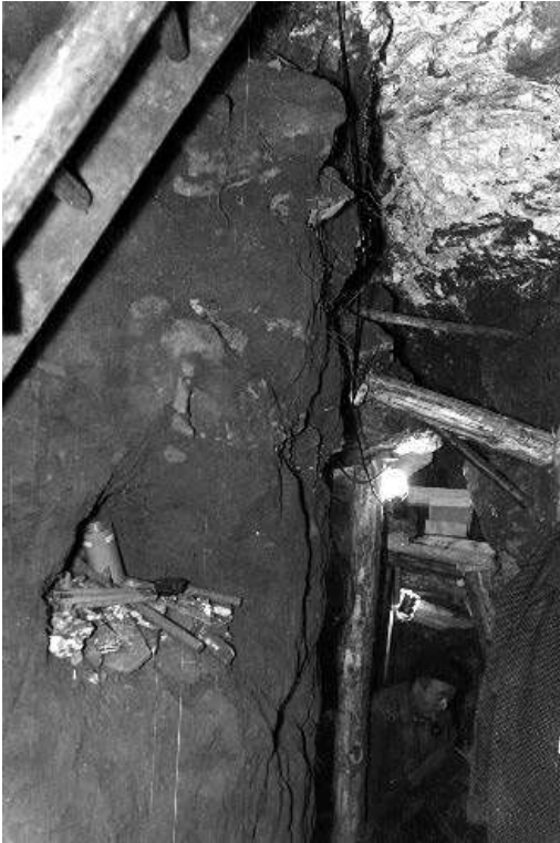
Figure 4 - View of the gallery dug by R. Constant after its shoring up.
