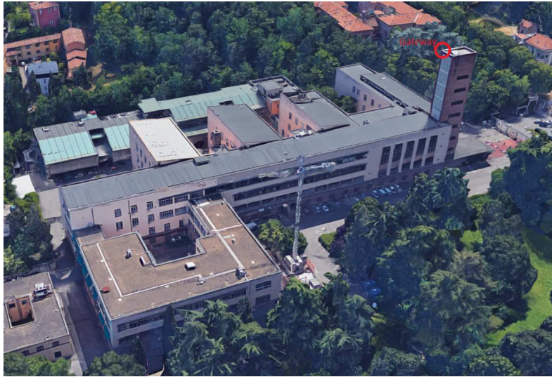
Fig. 5.2: 3D representation of the Engineering School of University of Bologna and LoRaWAN GW deployment.
