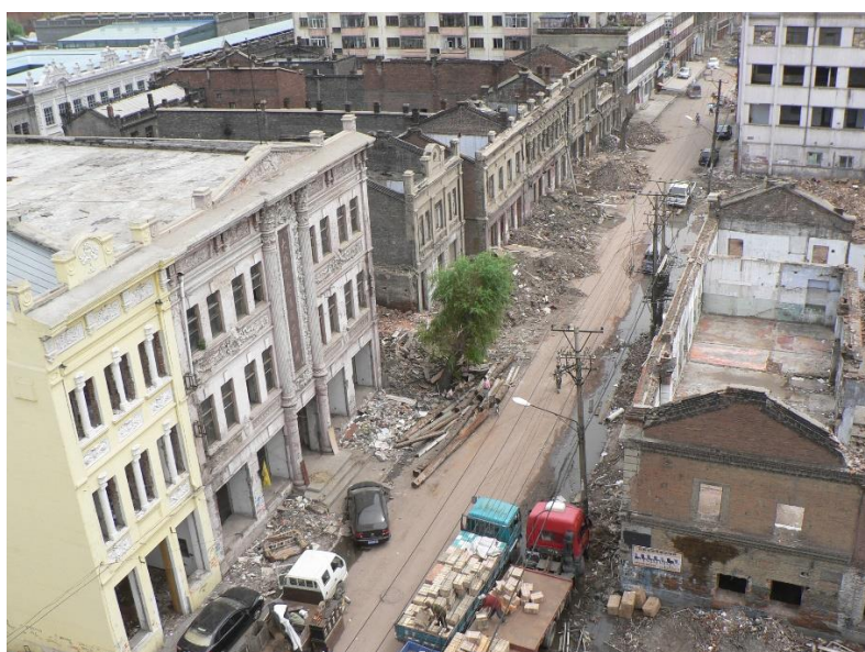
Figure 2. The Old Neighborhood under Renovation
