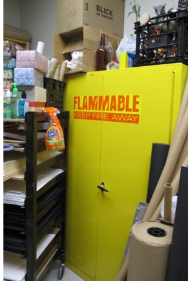
Figure 4.7.9 Site 4 blocked flame-resistant storage
