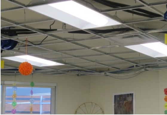
Figure 4.10.17. Site 18 exposed ceiling
