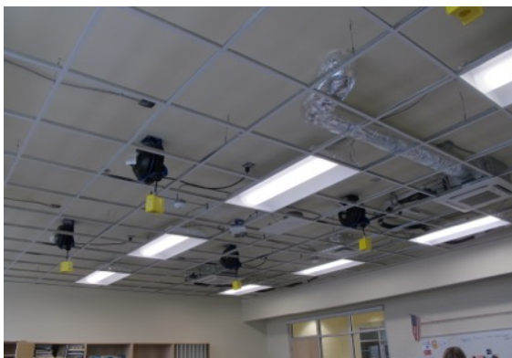
Figure 4.2.15. Site 18 open ceiling.
