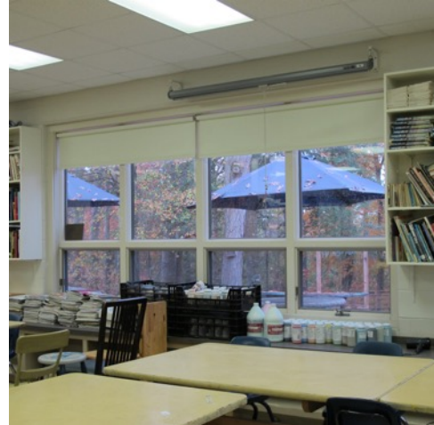
Figure 4.4.8. Site 12 screen installed in front of window.
