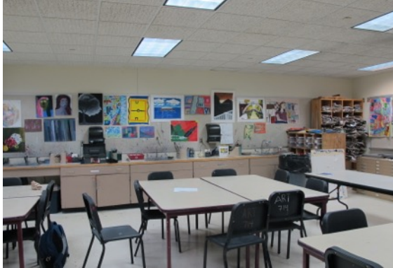
Figure 4.9.18. Site 9 classroom with no windows.
