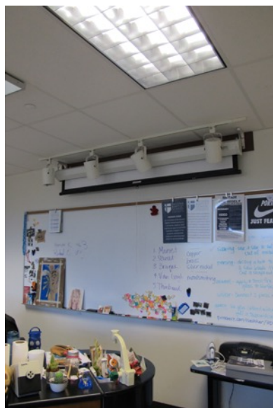
Figure 4.10.1. Site 3 track lighting installed over screen—or vice-versa.
