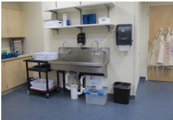
Figure 4.2.3. Site 18 ADA compliant sink?
