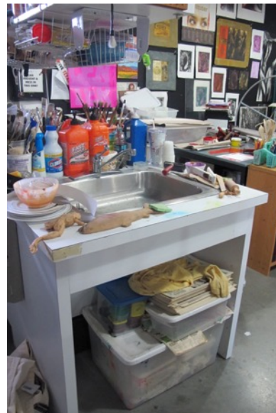
Figure 4.2.4. Site 11 ADA sink with blocked access.
