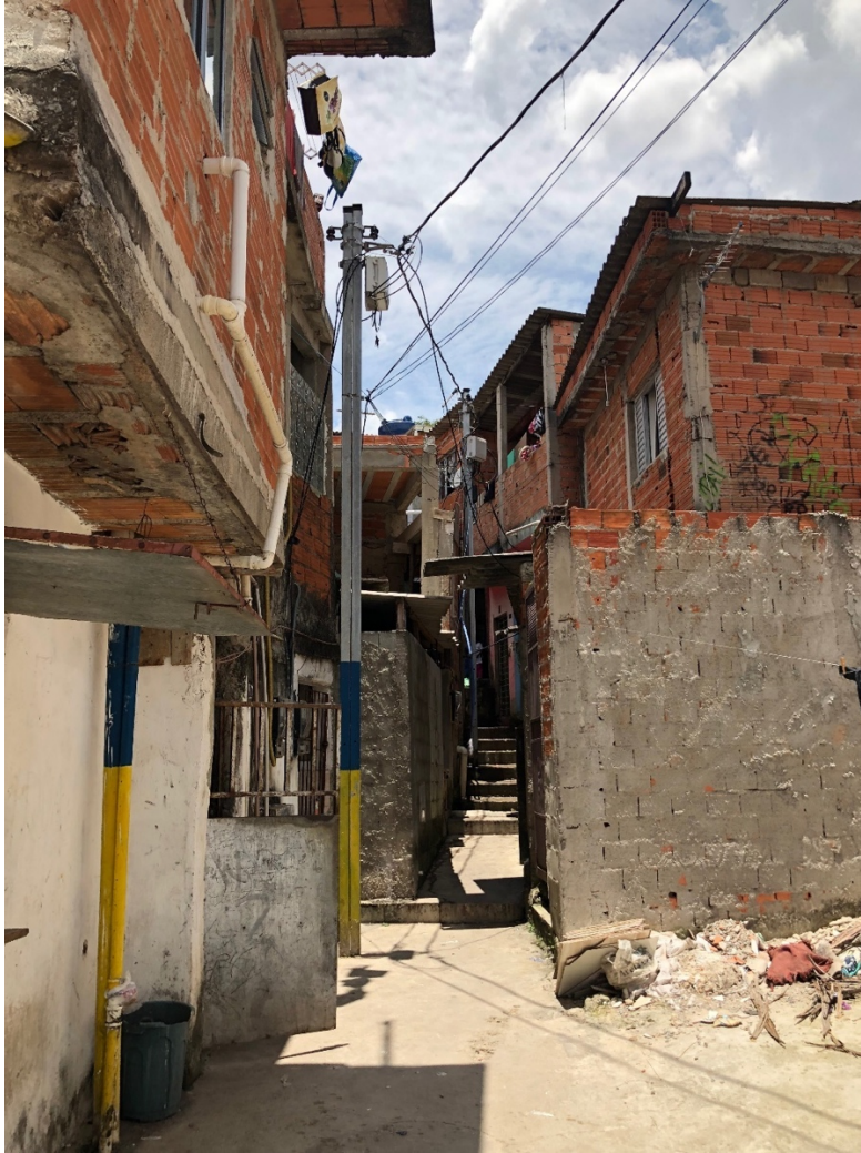
Figure 10. Alley in Sapé after completion of upgrading. Source: the author.
