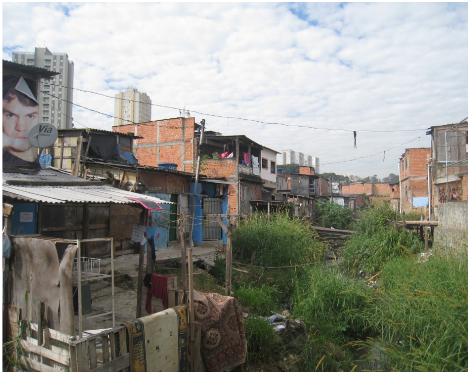
Figure 1. Sapé before the start of upgrading. Source: SEHAB.
