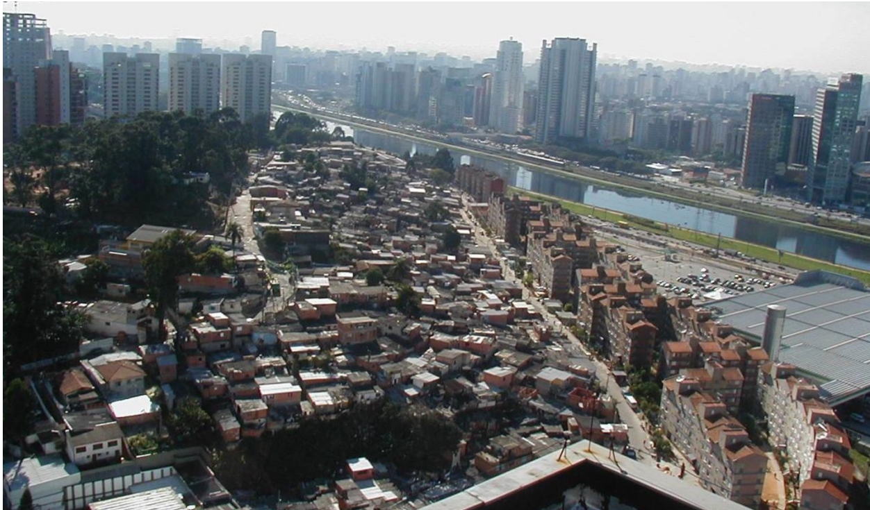
Figure 3. Real Parque before the start of upgrading. Source: SEHAB.
