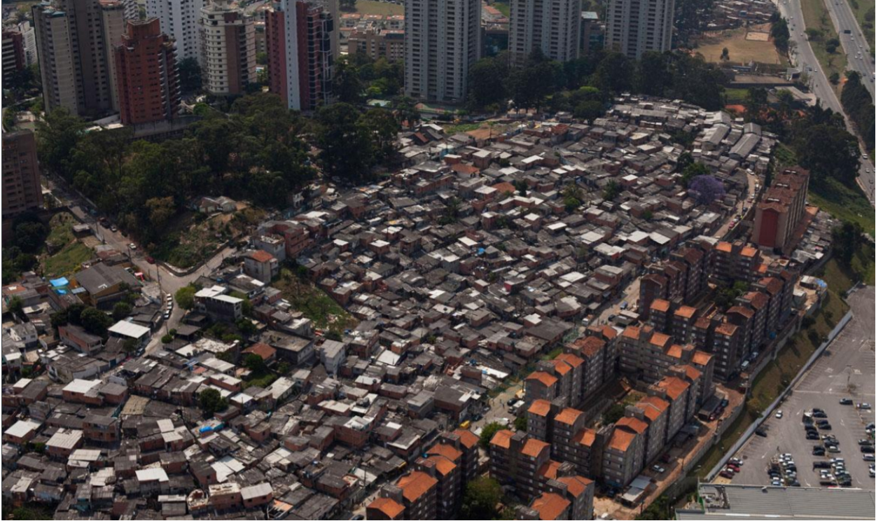
Figure 12. Real Parque before the upgrading works. Source: SEHAB.
