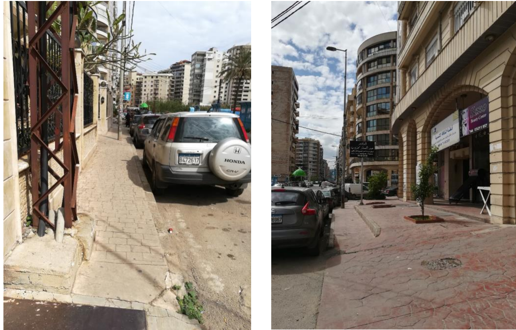
Figure 18: Interrupted Sidewalks in Dam w Farez
