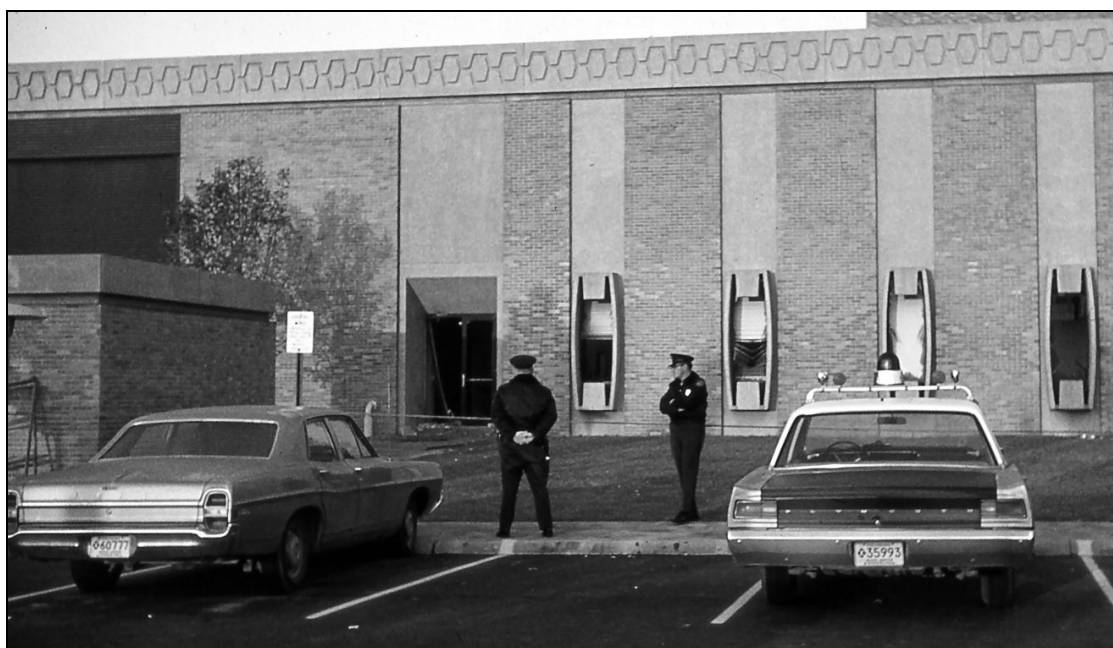
Figure 4: Bombed windows and doors of Emmett Leith's holography laboratory at the University of Michigan, October 1968. Courtesy C. Leonard.
