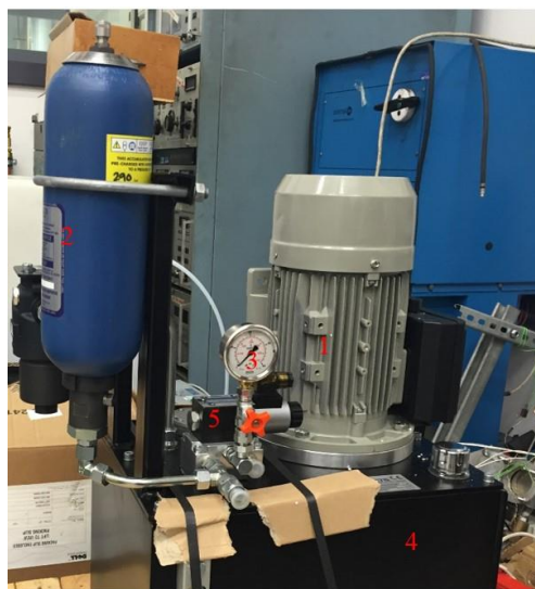
Figure 3.7: Picture of the large hydraulic pumping system for the actuator
