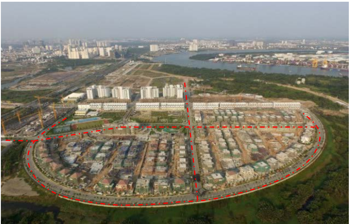
Figure 6. 1 Examples of transport development in following to urban development
