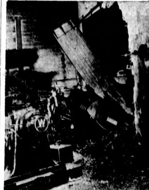
This is what a Pacific Electric Railway substation in Los Angeles, Calif., looked like after a 20-ton armature whirling at 750 r.p.m. tore loose from a generator. One piece of the armature was hurled through a six-inch reinforced concrete roof, but no one was injured. Herman Soder, rail employe, examines
