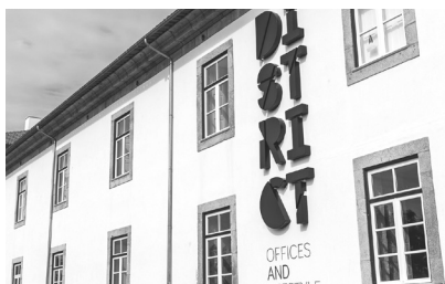
Fig. 3 Fachada do edifício District Offices and Lifestyle.
