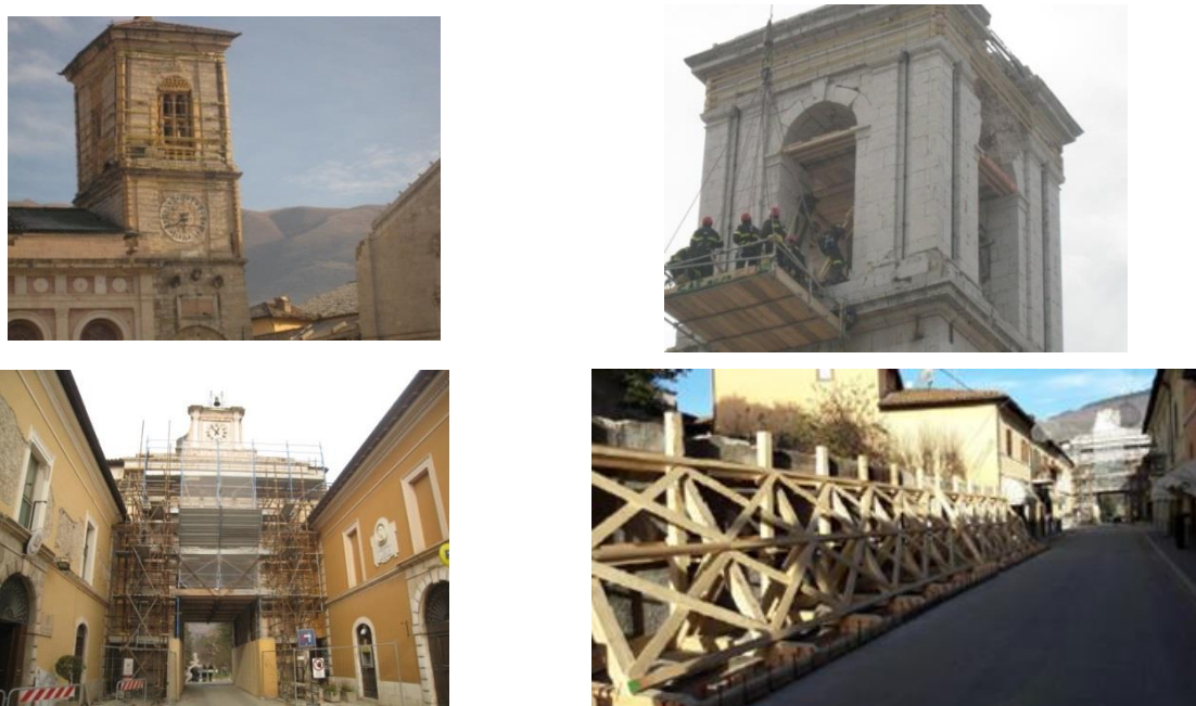
Figure 5 - Bracing of unstable constructions in Norcia by the fire brigades
