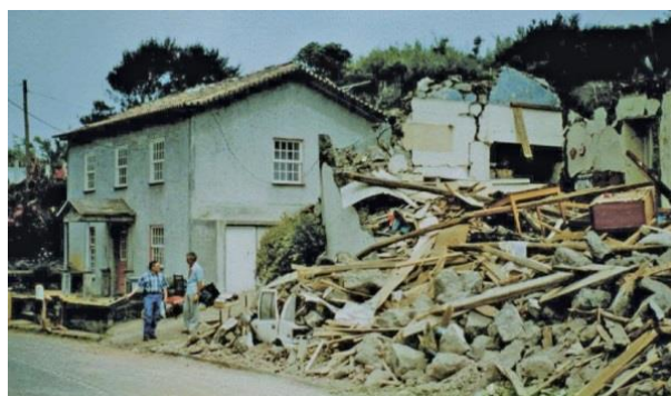
Figure 9. Difference of seismic performance between adjacent constructions
