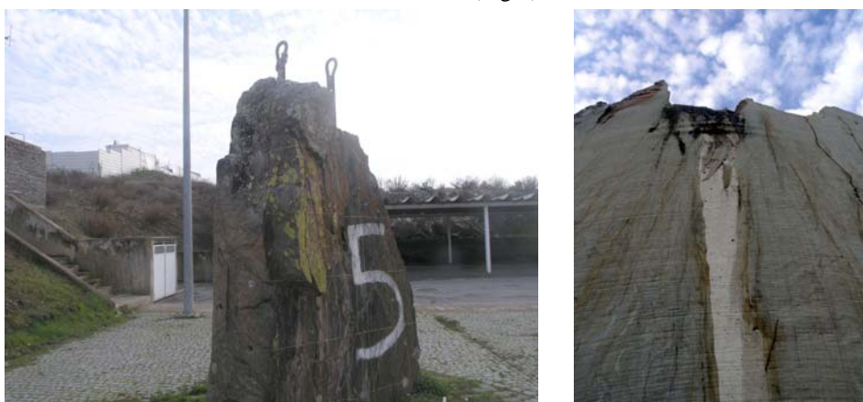
Figure 2 - Aspects of the translocated block. Notice on the right the saw cut surface and the mortar filling of the rock joint
