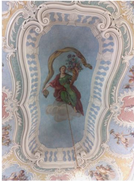
Figure 2 – The Grand Hall’s magnificent stuccoed ceiling
