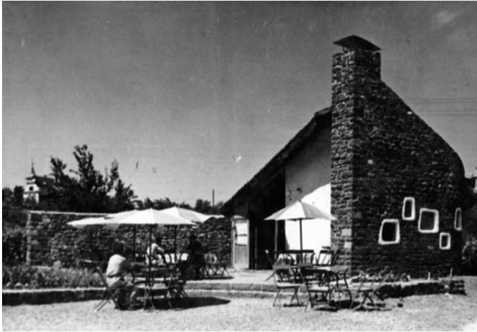
Figure 5. Wine pub in Badacsony. Architect: Ferenc Callmeyer. (IPARTERV photo archive, N° 3773)
