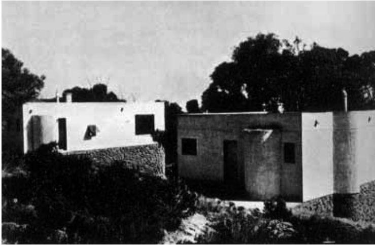
Figure 3. “Weekend” Houses in El Garraf – Barcelona. Background view of B and C Type. J. Luis Sert and J. Torres Clavé, architects. ( AC: Documentos de Actividad Contemporánea , nº 19, 1935: 39)
