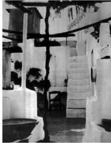
Figure 3. Courtyard in Vila Viçosa: photograph taken during the Survey's fieldwork. (in Popular Architecture in Portugal , third edition: 1988, vol.3, p.83)
