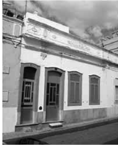
Figure 3. Viegas Pires house, Rua Sacadura Cabral 6 (Cerca do Júdice), Olhão, 2009. Unidentified designer. Planning permission obtained 21 st May 1917 (© Ricardo Agarez 2013)
