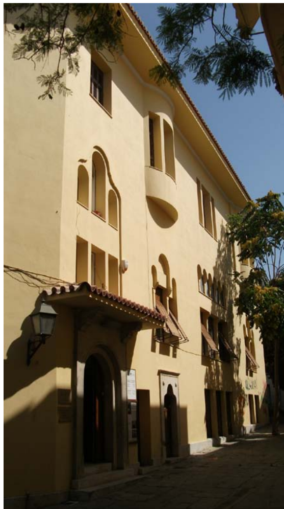
Figure 1. Aristotelis Zachos, Angeliki Hatzimichali's house, 1924-27
