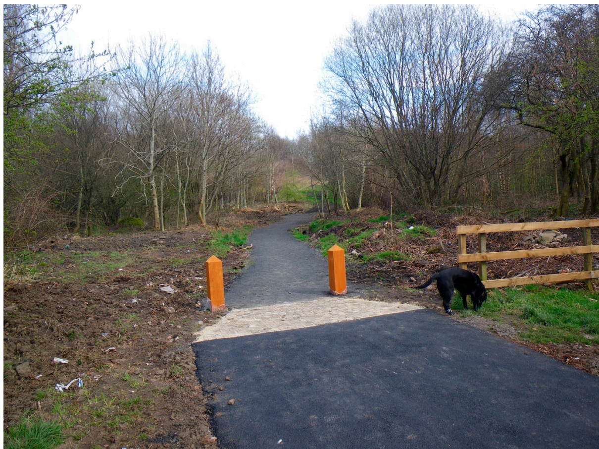
Figure 3. Typical woodland site post physical woodland intervention.
