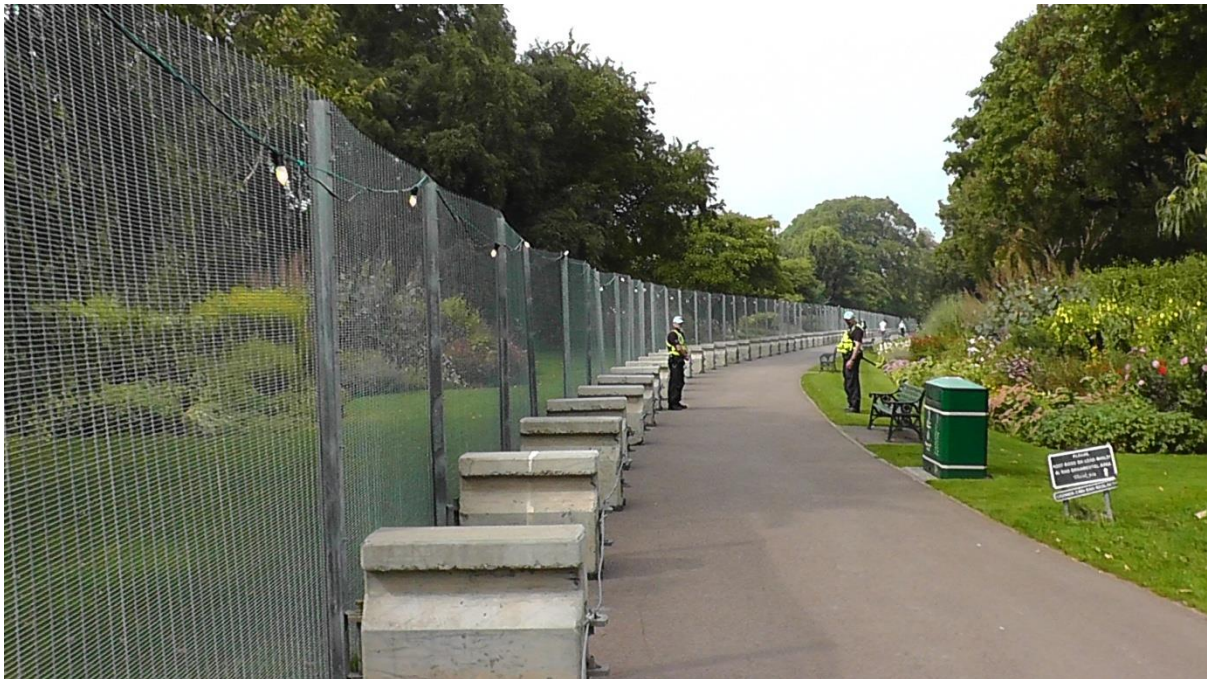
Picture 41 : Immoveable Objects: Steel Cable Fixings Inter-Linking Concrete Bollards Attached to Steel Fences and to Each Other
