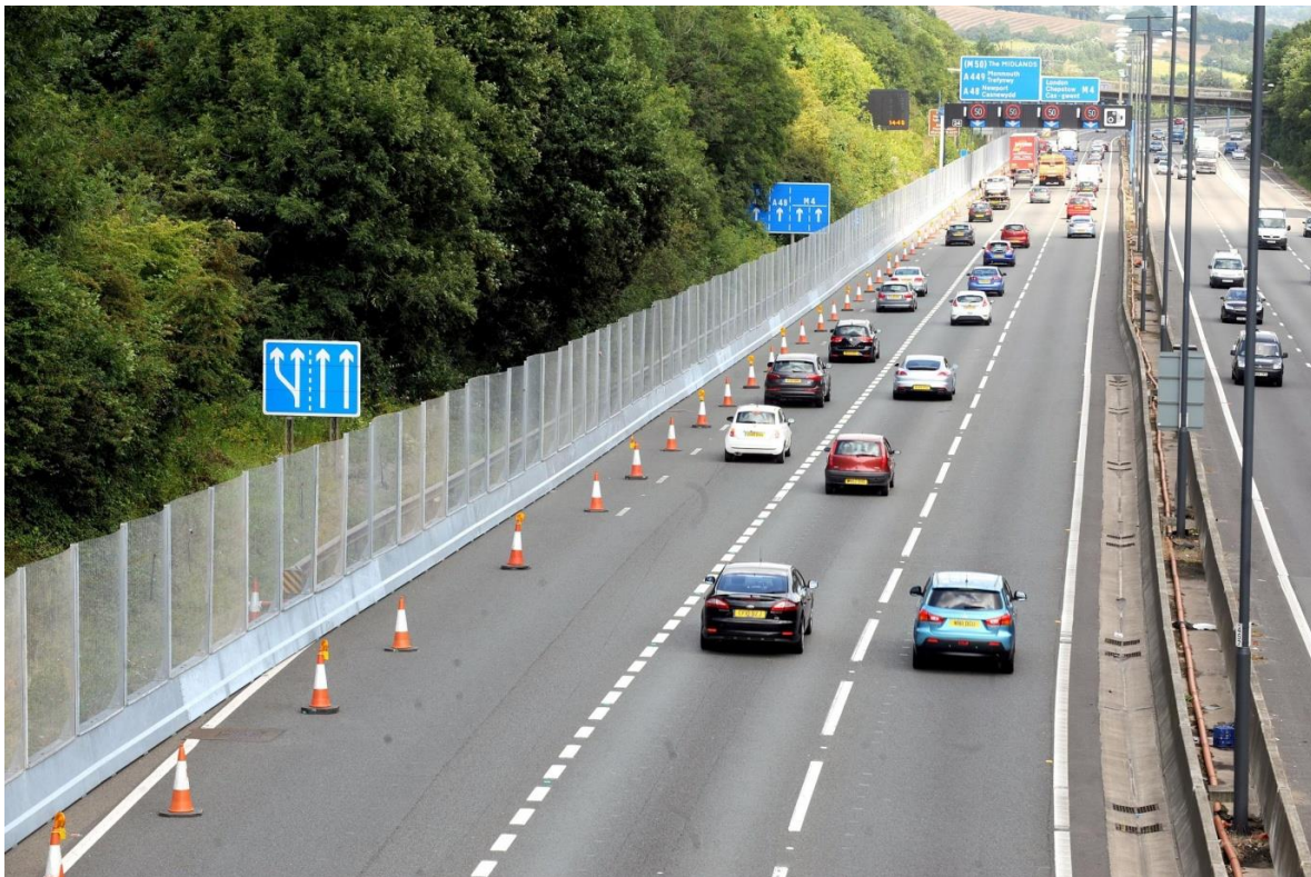
Picture 10: Part of the 'Ring of Steel' Fencing Bisecting Space Between the Summit Grounds and the M4 Motorway (Closing off One Lane of the M4)
