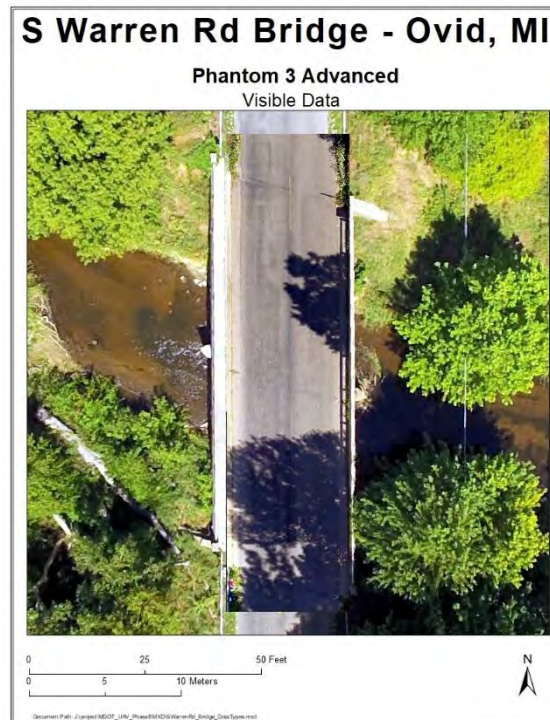
Figure 66: South Warren Road orthophoto.
