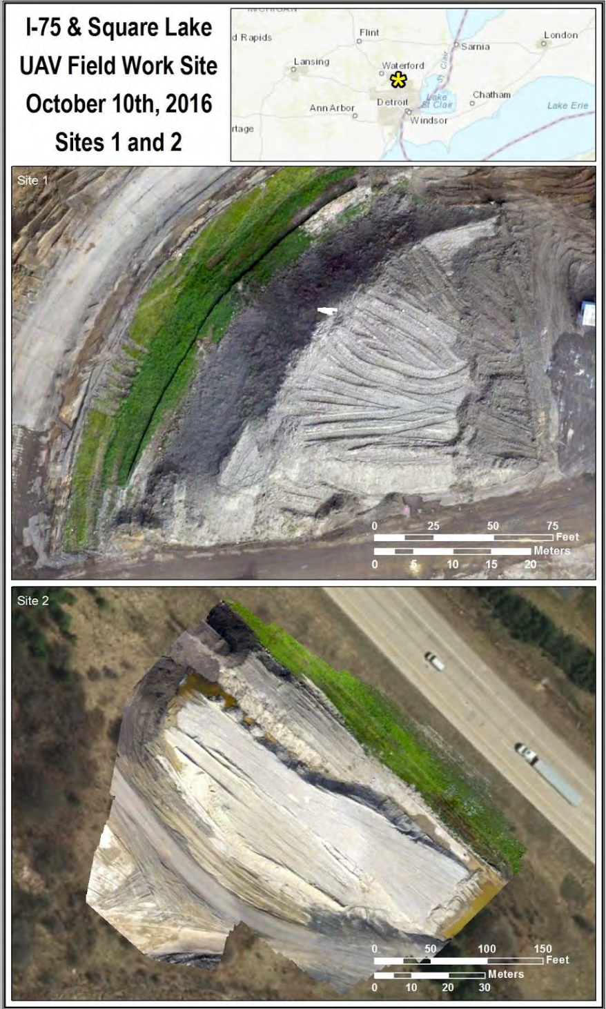
Figure 8: Orthophotos of two construction aggregate mounds at the I-75 Square Lake construction site collected with Bergen Hexacopter / Nikon D810 sensing combination.
