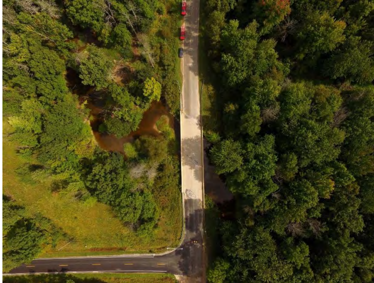
Figure 41: Example image from the Phantom 3A of the Gordonville Road bridge.
