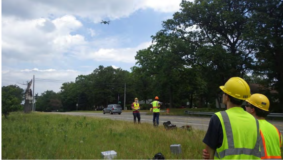
Figure 18: Collecting oblique imagery of the roadway for an overview map of the M-120/Holton Road corridor site with the Mavic Pro UAV.
