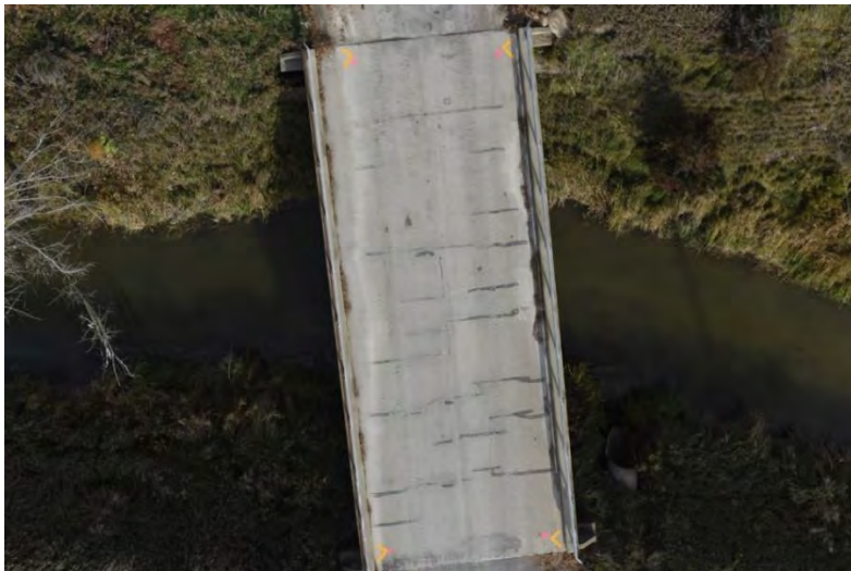
Figure 14: Nikon D810 image used for orthophoto and DEM creation for the Beyer Rd bridge.
