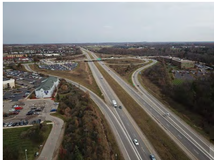
Figure 31: US-23 Road Corridor (looking north) as visible from a MTRI UAV.
