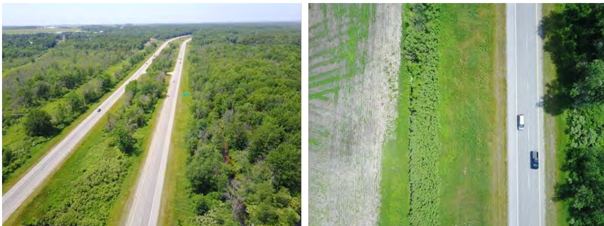
Figure 44: Two views of the US-31 / White River project location collected with the Mavic Pro UAV.
