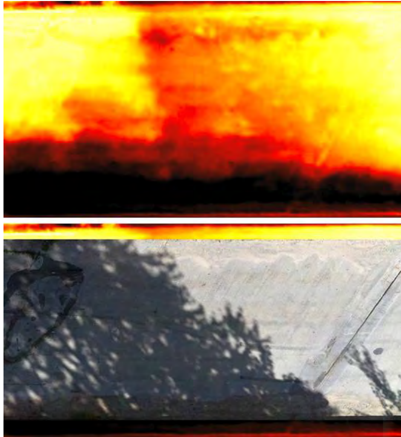
Figure 75: Comparison between the thermal (upper panel) and visible (lower panels) images at the Gordonville road test site. The presence of tree shadows, easily recognizable in the visible imagery (lower panel) mask the presence of potential thermal signatures related to delaminations (in the upper panel).
