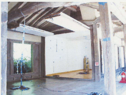
Pic.5 Ondol room with opened door
