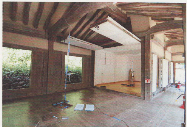
Pic.3 The Maru and Ondol room
