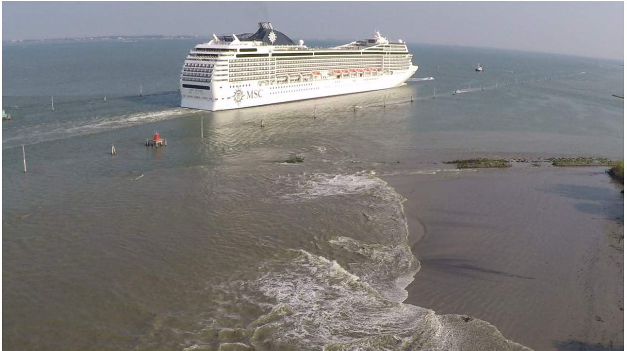
Fig 5. Aerial view of a cruise ship transit in the MMC. The depression wake exposes the collapsed materials of the original rip-rap revetment of the embankment at the southern end of the Cassa di Colmata B (CC-B). Image source: author's picture.
