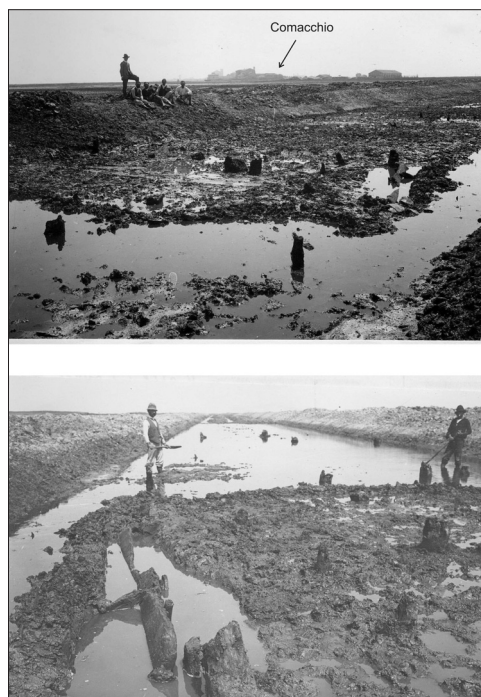
12. Comacchio: Valle Ponti. Photo made during the excavation works of the drain channel (30s of the 19 th century) with the recovery of wooden poles and planking pertinent to the port structures.
