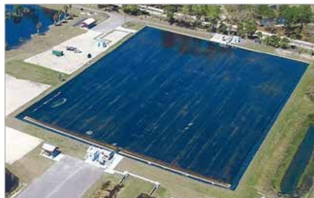
Figure 4. Aerial view of 10 MGD Egret Marsh Algal Turf Scrubber located in Indian River County, Florida. Photograph: Courtesy of HydroMentia, Inc.
