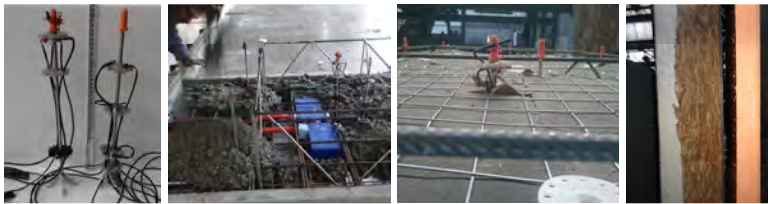
Figure 3. Installation of T-H sensors
