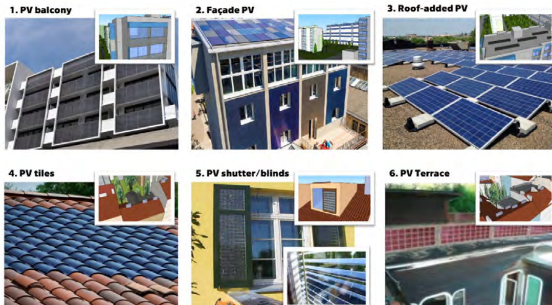
Figure 2. Examples of architecturally integrated PV systems in the two building blocks: (1) PV balconies. Source: Etsprojects; (2) Coloured PV-façade. Source: Swissinsol; (3) Roof-added PVs. Source: Cromwellsolar; (4) PV tiles. Source: Tradeford; (5) PV shutter and PV blinds. Source: COLT international, Solargaps; (6) PV terrace. Source: (López and Frontini, 2014).
