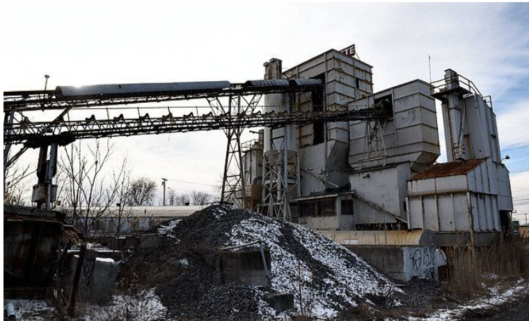
Clark Concrete, an old mixing plant, Solar and Van Rensselaer Sts. Ellen M.
