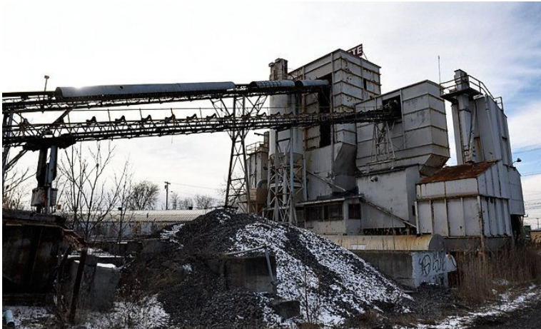
Clark Concrete, an old mixing plant, Solar and Van Rensselaer Sts. Ellen M.
