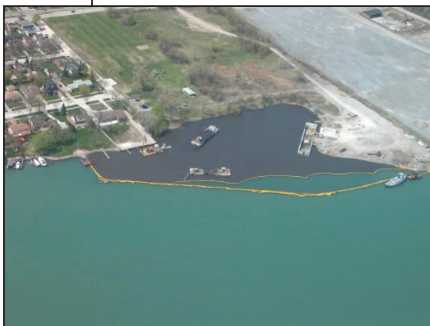
Figure 1. Black Lagoon sediment remediation project (Photo credit: Robert Burns, Detroit Riverkeeper).
