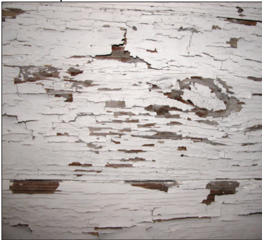
Figure 1. Deteriorated lead-based paint is one of the leading causes of lead poisoning in Detroit children (Photo credit: Emily Wilke).
