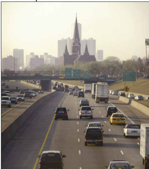
Figure 1. I-75 photo taken from the bridge on Ferry Street in Detroit, MI (Photo credit: Southeast Michigan Council of Governments).
