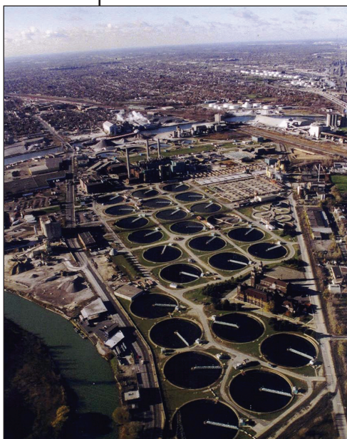
Figure 1. An aerial photograph of the Detroit Wastewater Treatment Plant ~ one of the largest in North America (Photo credit: Detroit Water and Sewerage Department).
