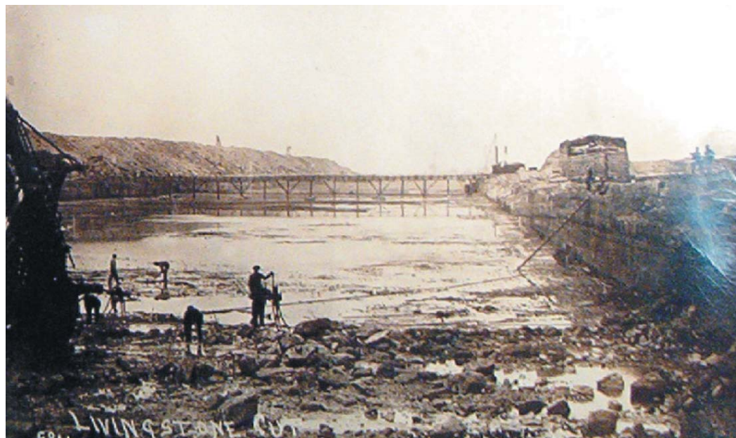
Figure 1B. Removal of historic limestone bedrock fish spawning habitat in the lower Detroit River during the 1907 Livingston Channel project (Source: Library of Congress).
