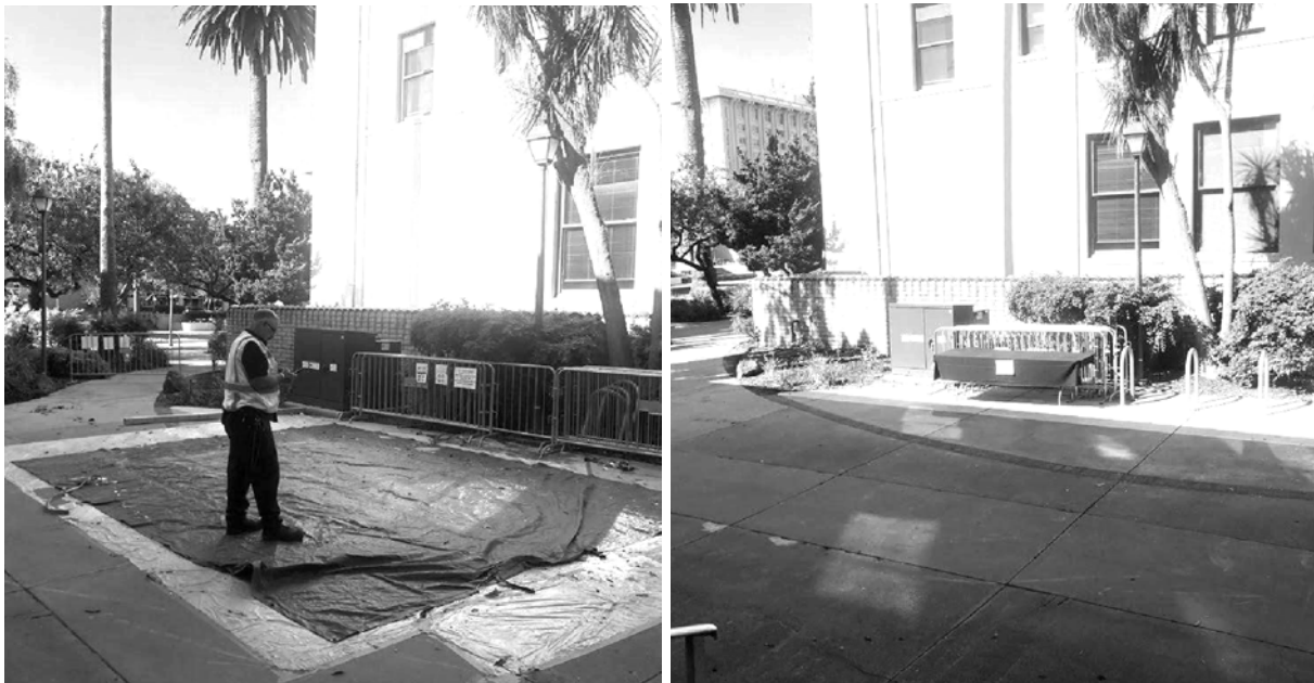
Figure H.20 - The conference site was cleared and cleaned.
