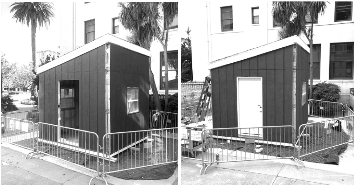
Figure H.12 - The exterior paint was completed (left) and the door hung (right).
