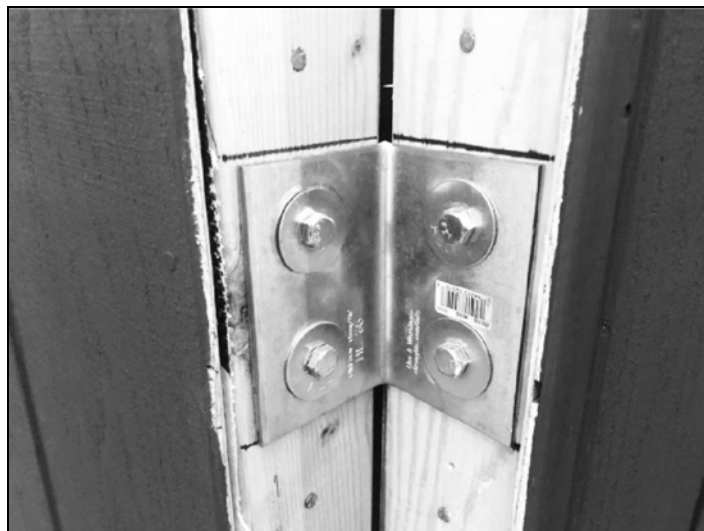
Figure 6.4 - The wall-to-wall corner connection installed on the cabin prototype.
