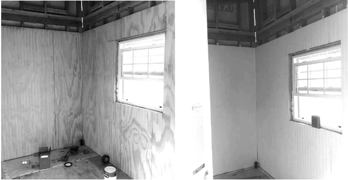
Figure H.13 - The interior plywood was hung (left) and painted (right).
