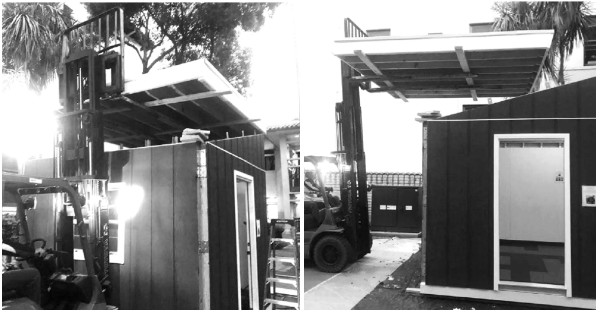
Figure H.16 - After the conference, the house was dismantled, starting with the roof.
