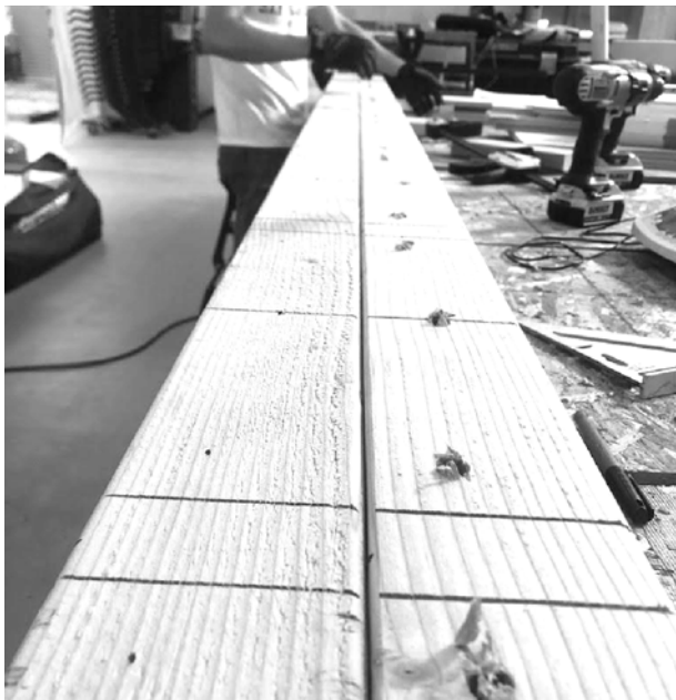
Figure H.2 -. Wall end studs, top plates, and sole plates had to be prepared for connections (T-nut installation and hole drilling).
