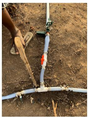
*Figure 12:* The connection of values to the hose at a T-joint using male adapters. Values can be seen on all three sides of the T-joint.
