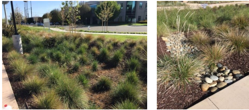
Figure 42. Municipal Site 6 (2016) with an infiltration rate of 8.2 in/hr., and a total criteria score of 24 (Photo by author).
