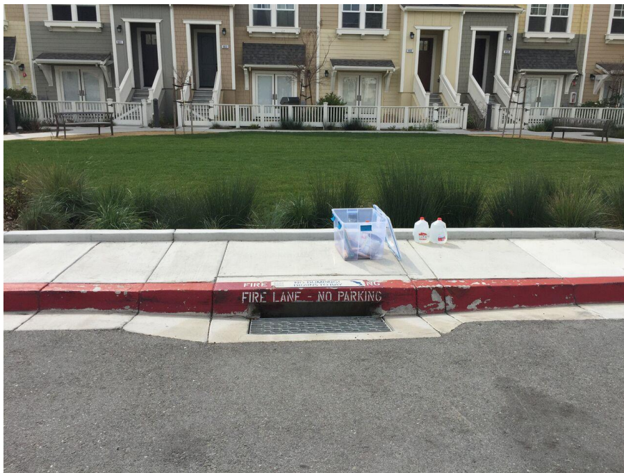
Figure 9. Municipal Site 3 storm sewer drain (Infiltration Rate: 40.0 in/hr.) (Photo by author).
