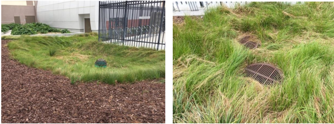
Figure 38. Campus Site 9 (2015) with an infiltration rate of 8.8 in/hr., and a total criteria score of 23 (Photo by author).
