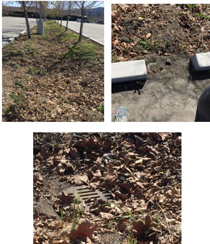
Figure 33. Campus Site 2 (2014) with an infiltration rate of 62.1 in/hr., and total criteria score of 22 (Photo by author).
