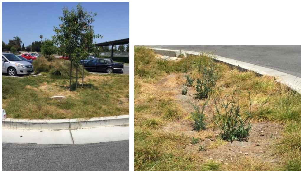
Figure 49. Municipal Site 36 (2014) with an infiltration rate of 10.0 in/hr., and a total criteria score of 20 Total Criteria Score 20 (Photo by author).
