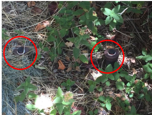
Figure 11. Site C12 sprinkler heads (Infiltration Rate: 19.1 in/hr.) (Photo by author).
