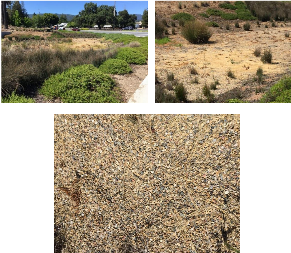
Figure 34. Campus Site 11 (2013) with an infiltration rate of 52.9 in/hr., and a total criteria score of 21 (Photo by author).
