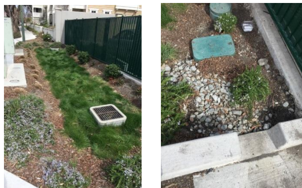
Figure 41. Municipal Site 5 (2016) with an infiltration rate of 6.5 in/hr., and a total criteria score of 23 (Photo by author).
