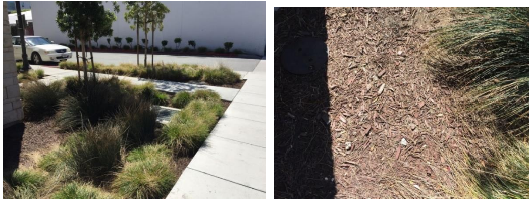
Figure 36. Municipal Site 12 (2013) with an infiltration rate of 61 in/hr., and a total criteria score of 25 (Photo by author).
