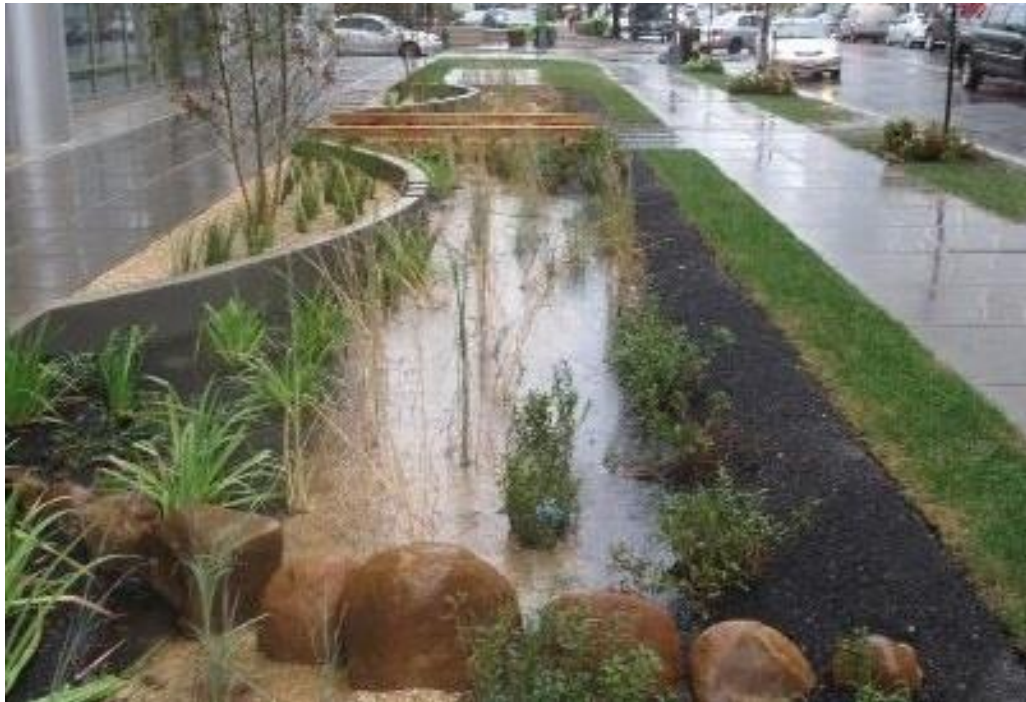
Figure 3. Bioswale along a city street in California (Mackie, 2017). Reprinted with permission.
