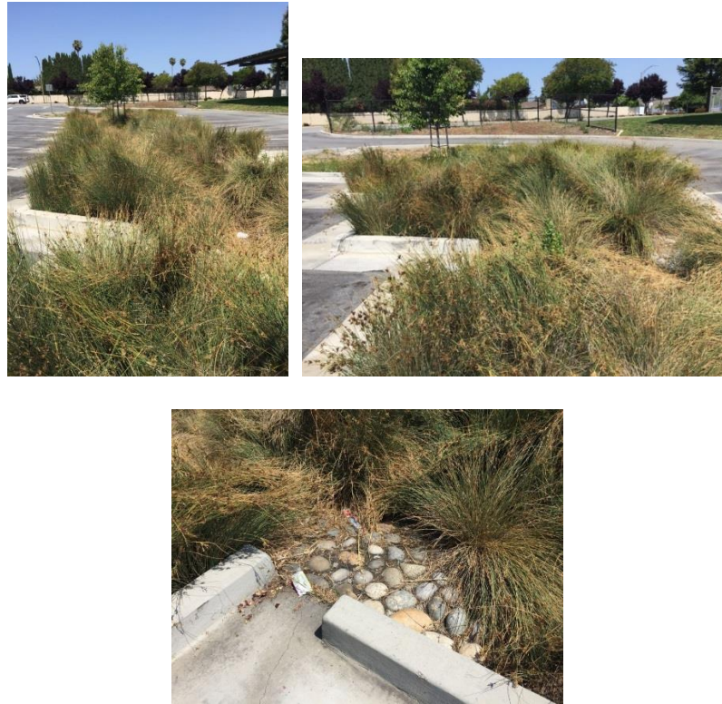
Figure 48. Municipal Site 35 (2014) with an infiltration rate of 7.8 in/hr., and a total criteria score of 21 (Photo by author).
