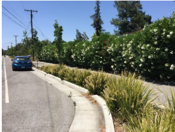
Figure 47. Municipal Site 27 (2011) with an infiltration rate of 10.0 in/hr., and a total criteria score of 23 (Photo by author).
