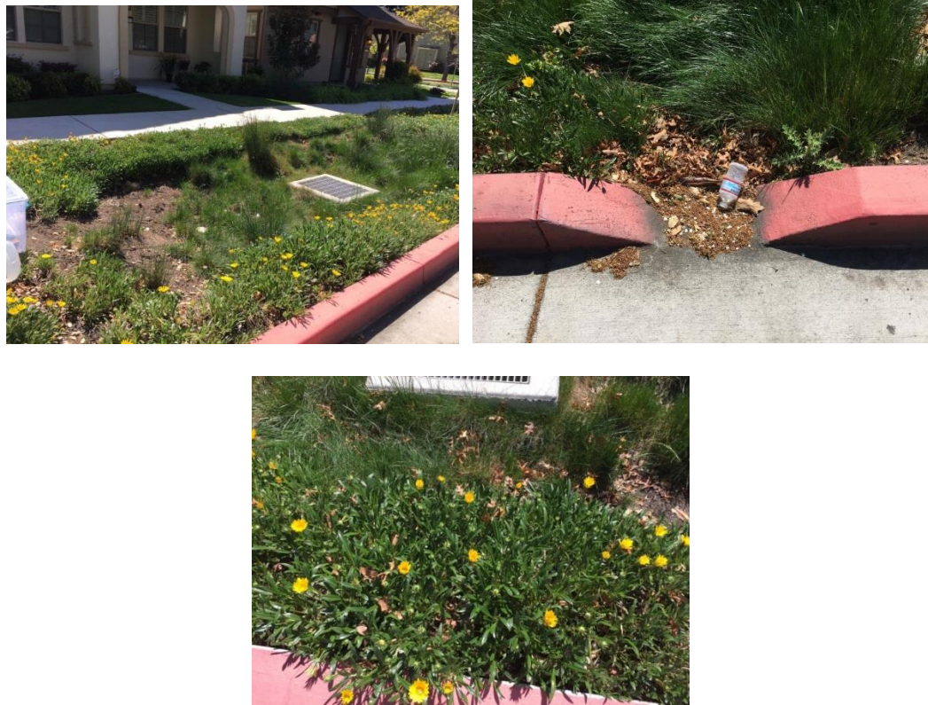
Figure 35. Municipal Site 10 (2015) with a infiltration rate of 40 in/hr., and a total criteria score of 22 (Photo by author).
