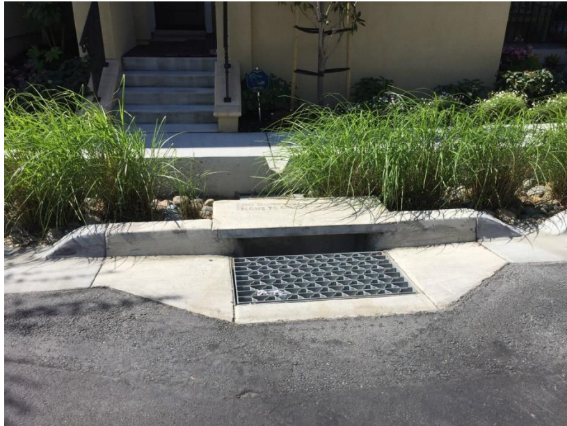
Figure 10. Municipal Site 11 storm drain (Infiltration Rate: 5.7 in/hr.) (Photo by author).
