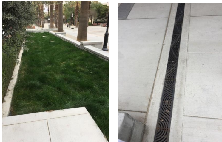
Figure 30. Campus Site 5, with a total criteria score of 27, and an infiltration rate of 27.7 in/hr. (Photo by author).
