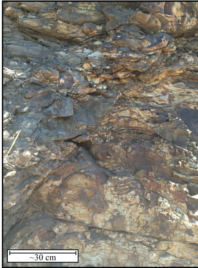
Figure 9. Outcrop showing a fault and fracturing in the Ruby Creek-Windmill Point area.
