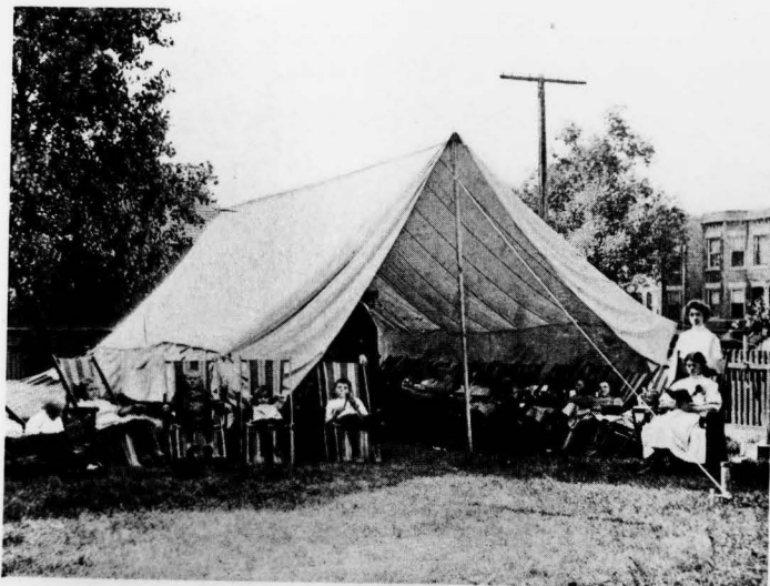
The classroom tent of the first Chicago school
