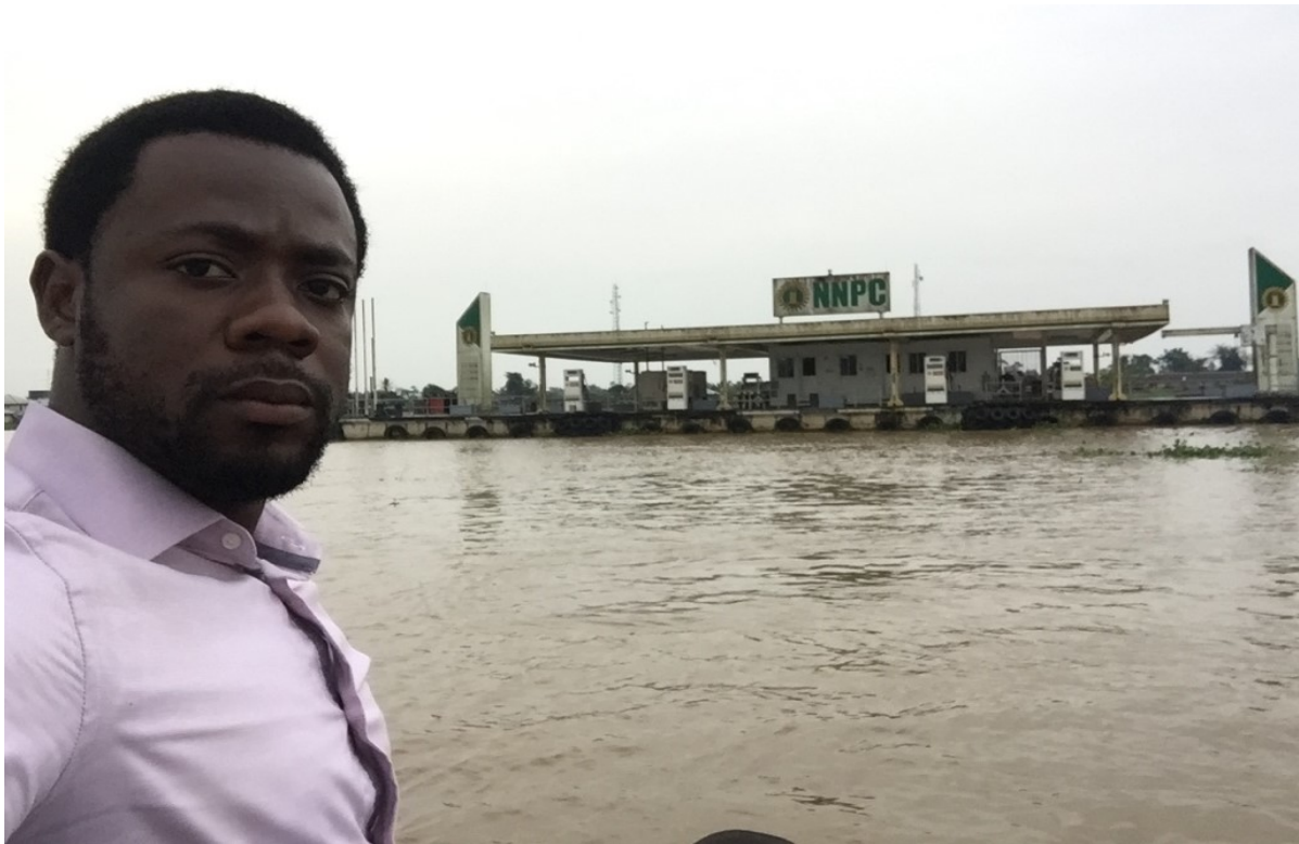
Figure 7-16 a non-functioning NNPC floating filling station in Osiama Creek and Ogubiri River
