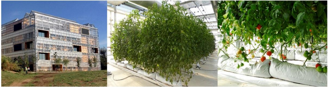
Figure 1. ICTA-ICP building with the i-RTG on the top (left), the i-RTG with a crop in the vegetative stage (middle), and the i-RTG with a crop in the harvesting stage (right).
