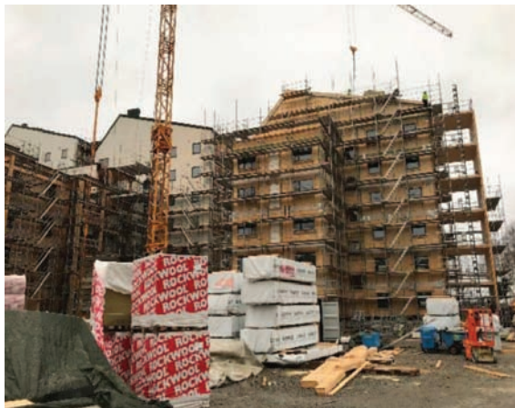
Figure 1. Wooden buildings are built without weather protection.
