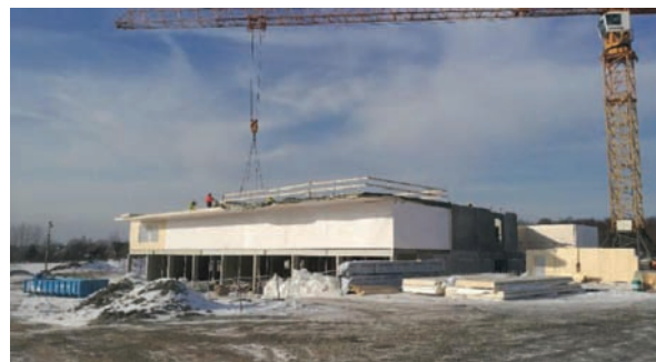
Figure 1. CLT floor elements covered by packaging film and stored on-site before installation process (left). Overall view of CLT element installation process (right).
