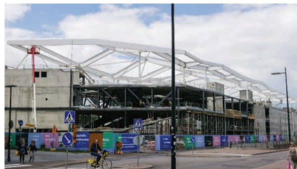
Figure 1. Element producing and lifting with the cranes (left). Helsinki Central Library concrete and metal frame (right)
