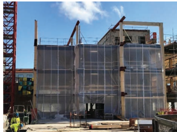
Figure 2. Office building with CLT-frame is built without weather protection.
