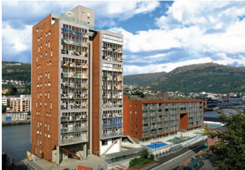
Figure 12. The world's tallest timber building, Bergen, Norway (2015).
