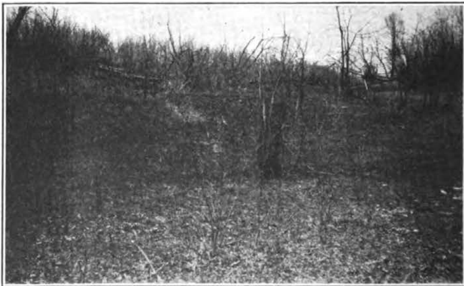
FIG. 24.—A washout made by the flood of 1898. It has not only become completely resodded but trees are thriving in what was once the soilless gravel bottom. Location H, figure 16.
