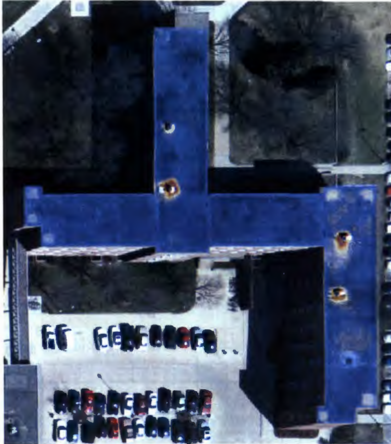
Figure 16. Thermal data overlay, Rider Hall.
