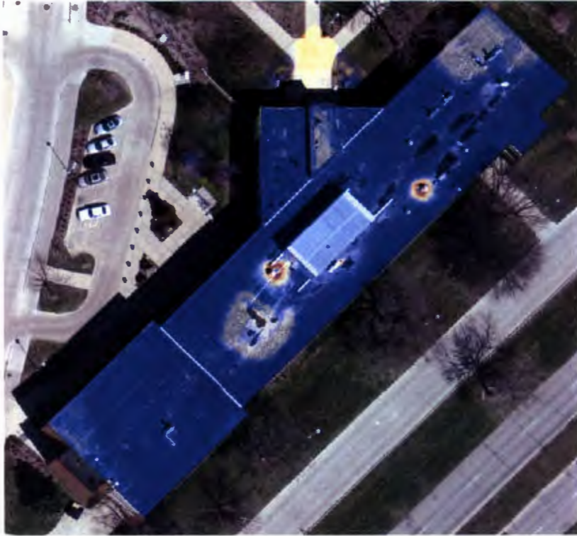
Figure 15. Thermal data overlay, Latham Hall.
