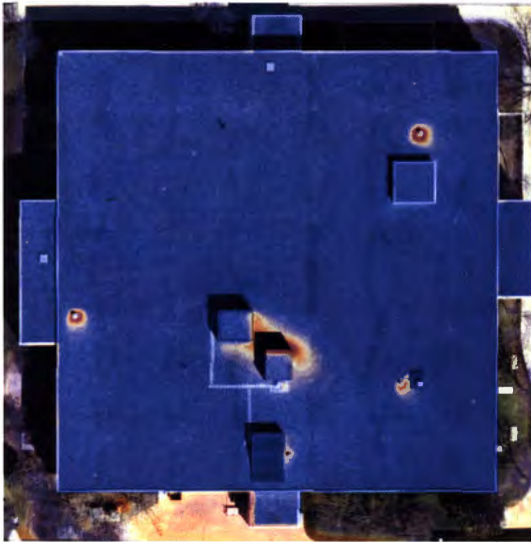
Figure 12. Thermal data overlay, Rod Library.
